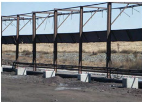
Construction of support beam platforms
