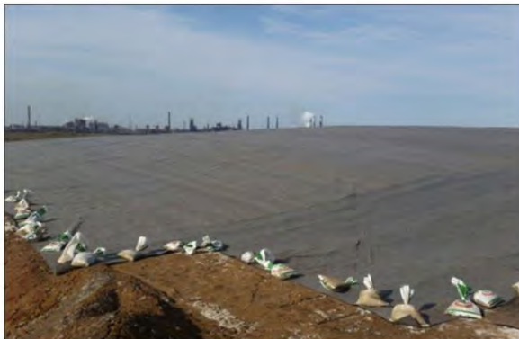
Filled Salt Cell covered with 2 x 150 mm clay layers compacted (beneath the black liner) and 1.5 mm HDPE liner
