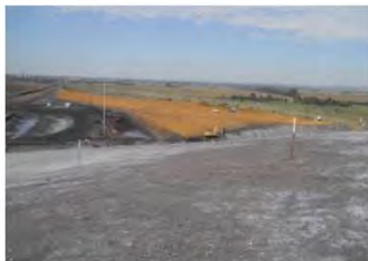
Before Capping at phase 2 - near tip station
