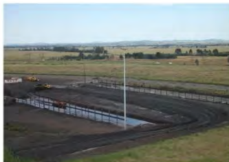
After Capping at phase 2 - near tip station
