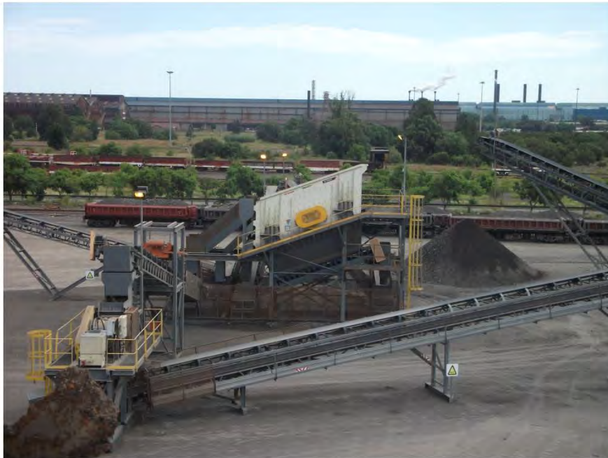
Lined operational area
