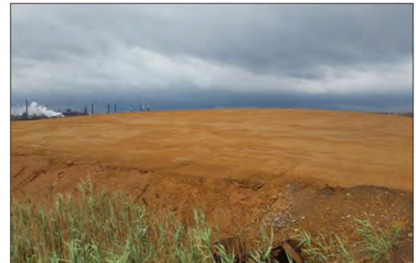
Salt Cell covered with top soil awaiting hydro-seeding
