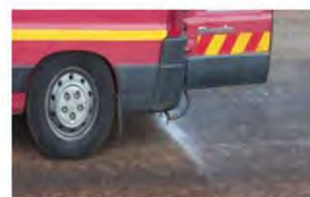
Sprayer system used to spray product onto the road
