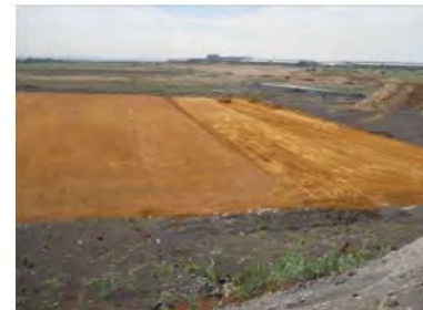
Domestic site: Clay liner layer
