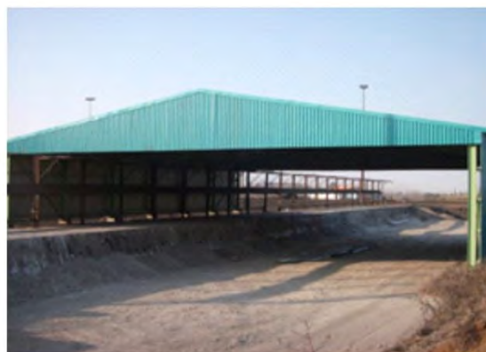
Completed structure including steel roof and steel side covers
