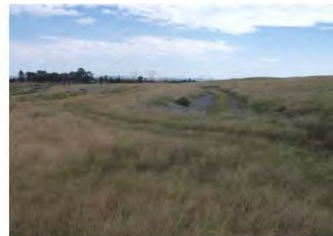
After Capping at phase 2 - drainage channel
