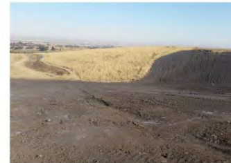
Before Capping at phase 3 - drainage channel
