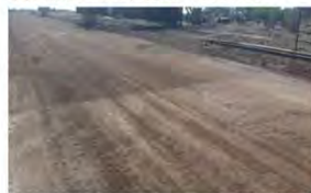
Clear distinction between treated and untreated section of roads
