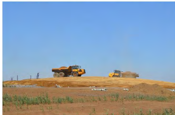
Salt Cell being covered with 200 mm top soil for hydro seeding purposes
