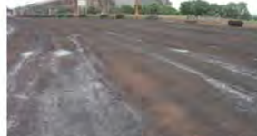
Road directly after product application
