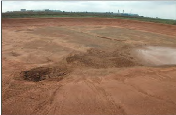
Salt Cell after earth moving work and shaping has been completed
