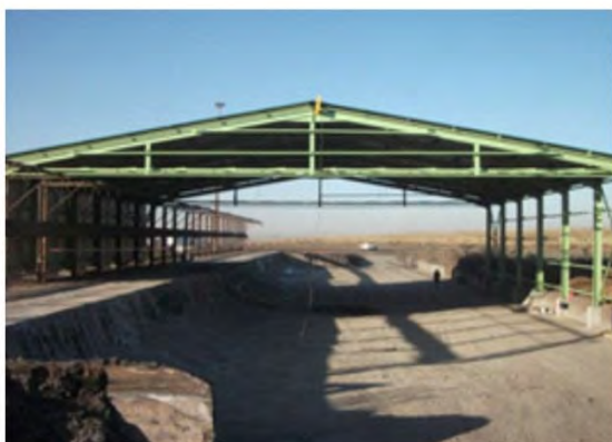
Installation of steel roof completed
