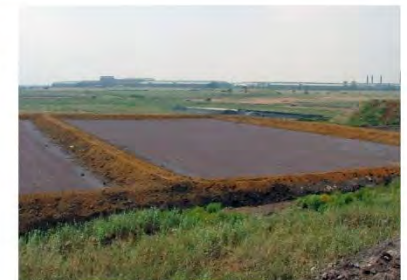
Domestic site: Stone protection layer and drainage collection channel
