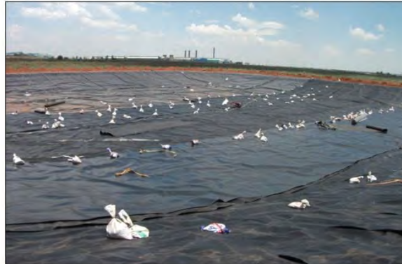
2 x Cusped geosynthetic drainage layers followed by 3 x 1.5 mm HDPE (High Density Polyethylene) liners being installed
