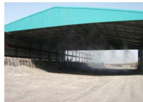
Sprayer system in operation to reduce fugitive emissions
