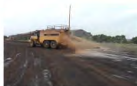
Product being applied to the road
