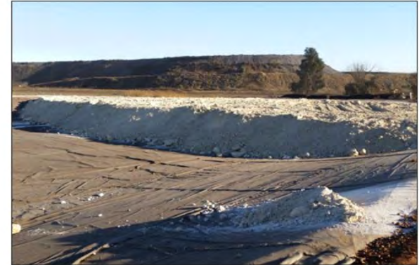
Salt being deposited into the lined Salt Cell
