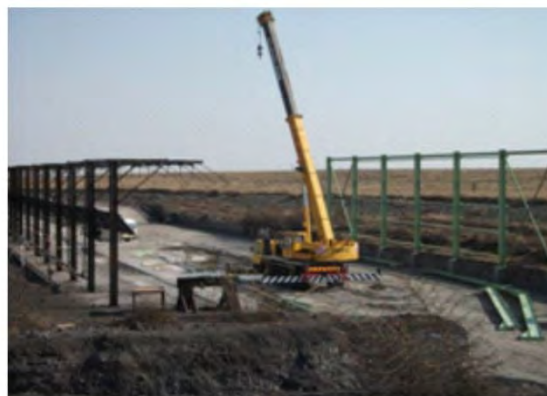
Construction of steel support beams for the roof
