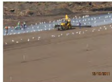
Domestic site: Laying of plastic liner
