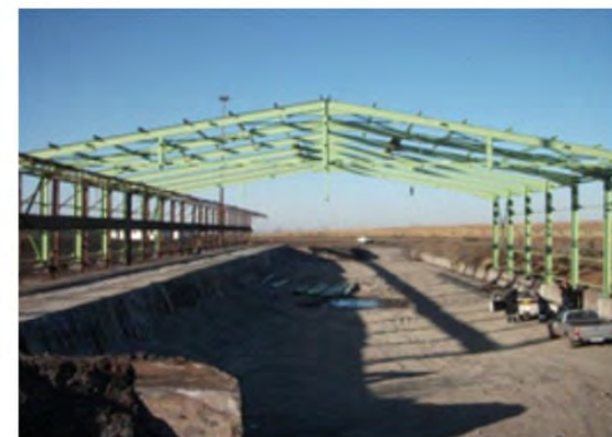
Completed steel frame
