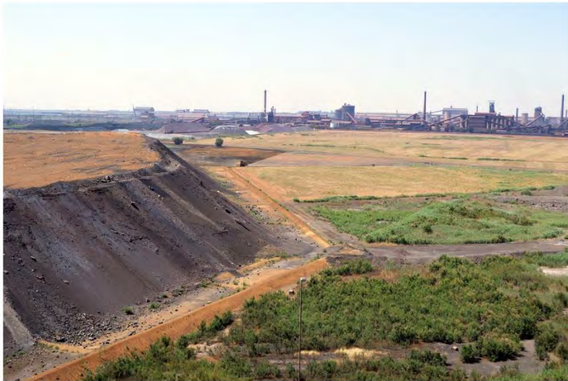
Operation of Dry Metallurgical waste site (G:L:B+)
