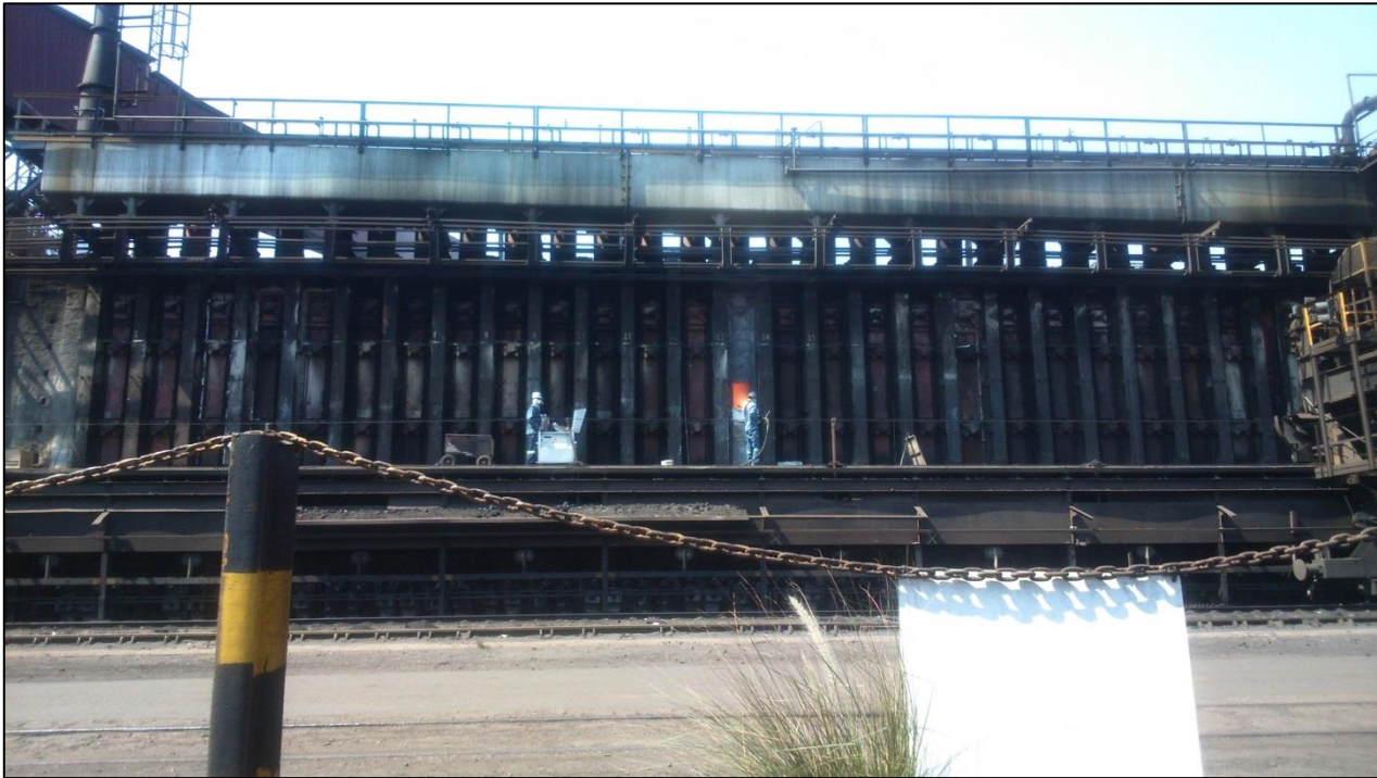
Figure 19: On-going coke oven door maintenance
